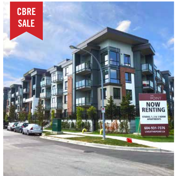
The Point Apartments: 5393 201st Street, Langley, BC Sold by the National Apartment Group BC | CBRE Limited June 2019; $39,000,000
